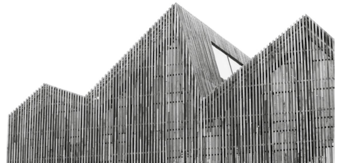
04. Facciata in palancole in legno del Museum Kaap Skil dei Mecanoo a Texel | Façade made of sawn sheet piles of Mecanoo’s Museum Kaap Skil in Texel. Chiara Scanagatta
